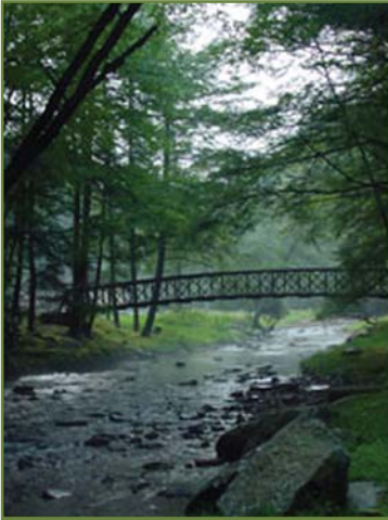
Foot Bridge over Tom's Run, Cook Forest
